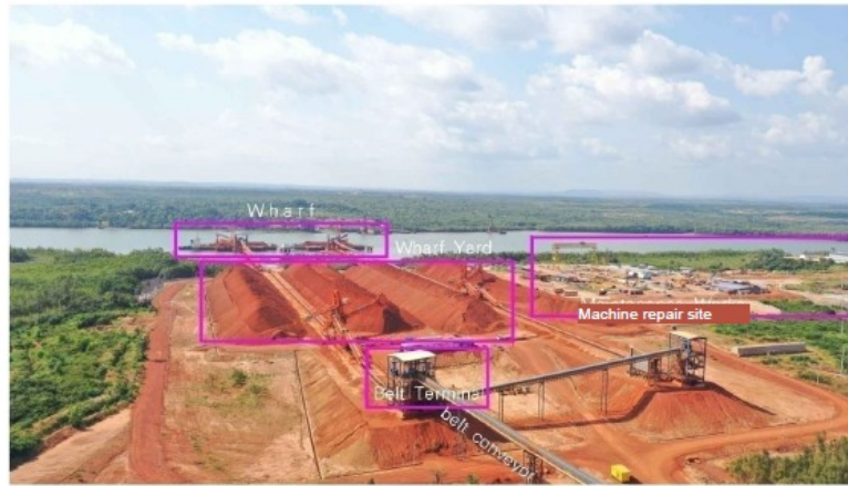
Fig. 5-3 Wharf and Wharf Yard in Boffa Mine
