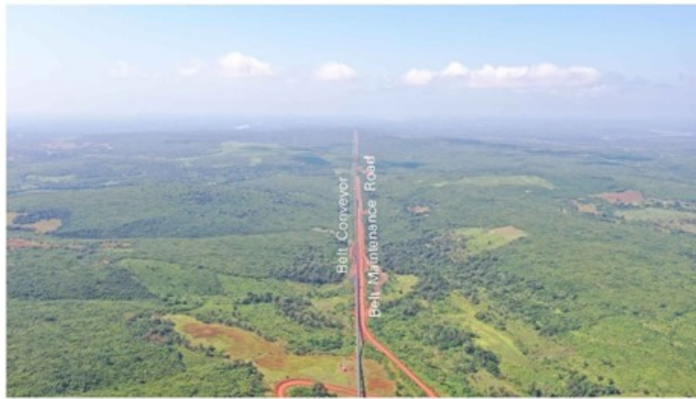
Fig. 15-4 Belt Conveyor and its Maintenance Road
