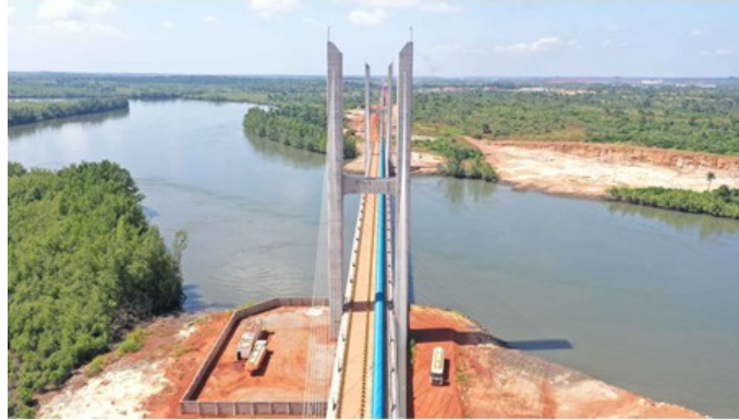
Fig. 15-5 The Cable-Stayed Bridge Crossing the Fatale River
