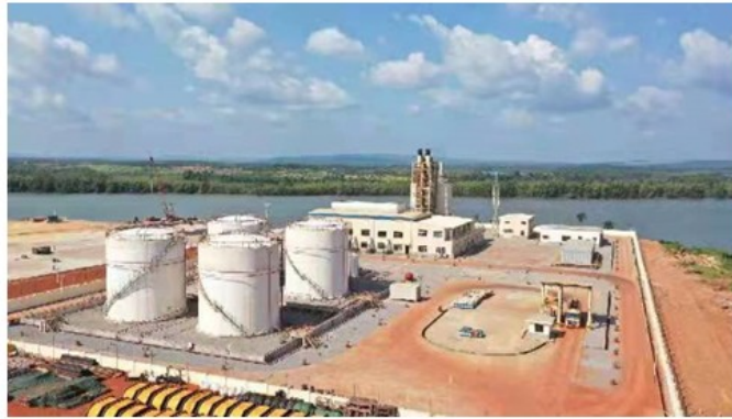
Fig. 15-7 Heavy Oil Power Station
